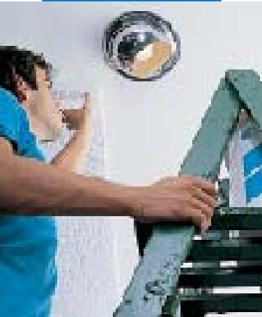
Installing an expanded-polystyrene ceiling
