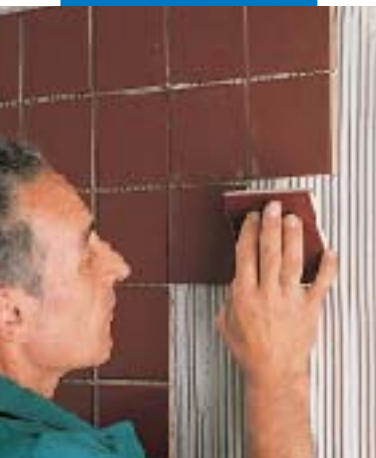
Tiling on gypsum plaster
