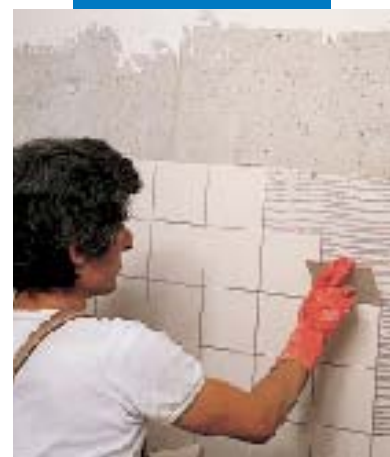
Tiling on reinforced-concrete walls
