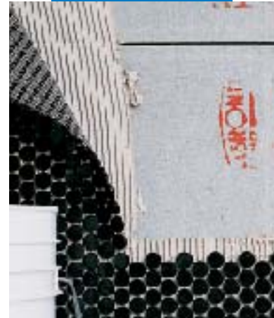
Tiling on fibre-cement
