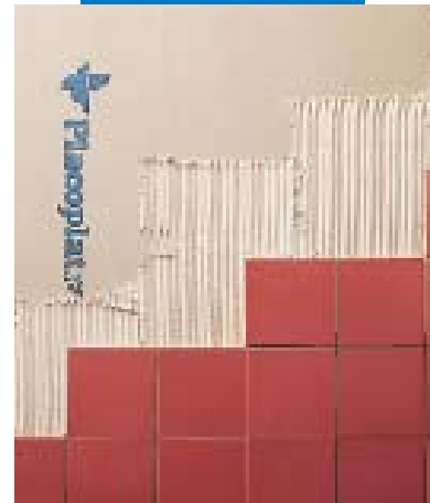
Tiling on gypsum board
