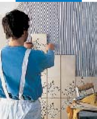
Tiling on ordinary plaster
