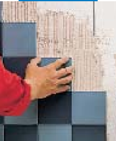
Tiling on expanded polystyrene
